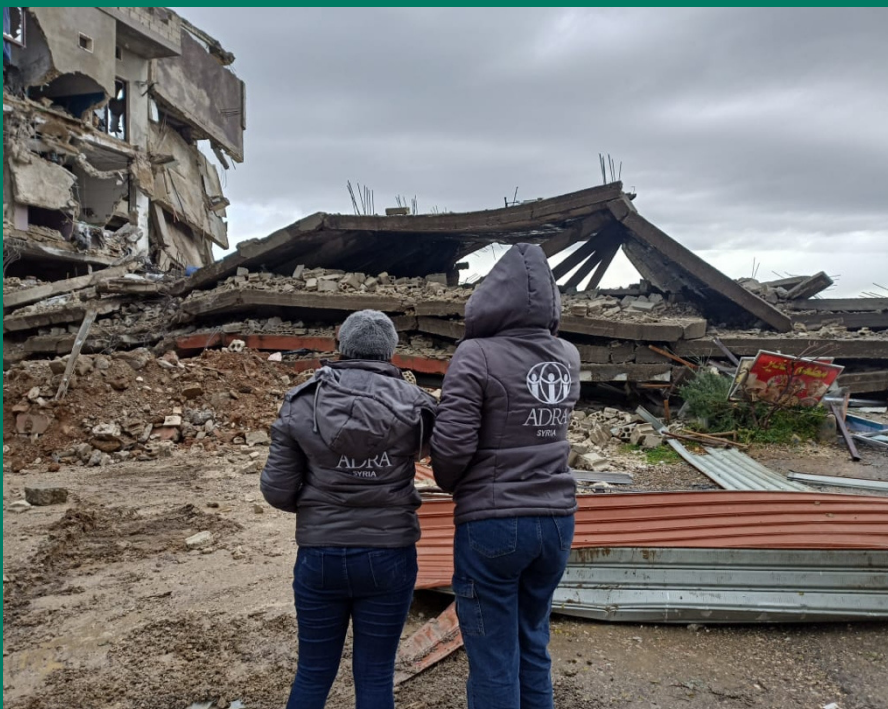
ADRA team in rural Latakia assessing the situation after the earthquake, February 2023
