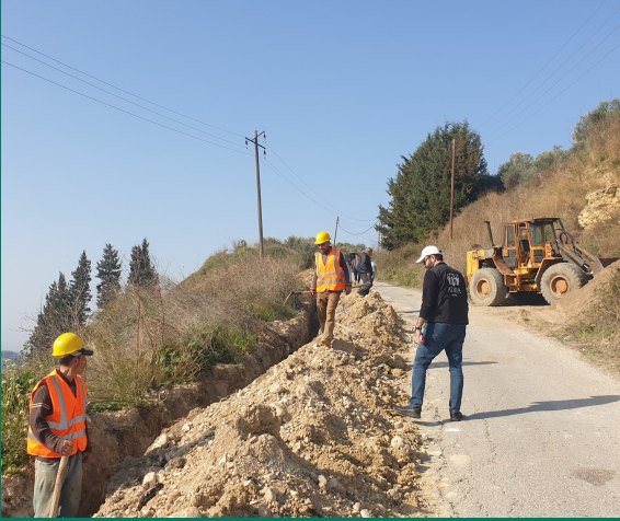
Ongoing rehabilitation work of underground pipes
