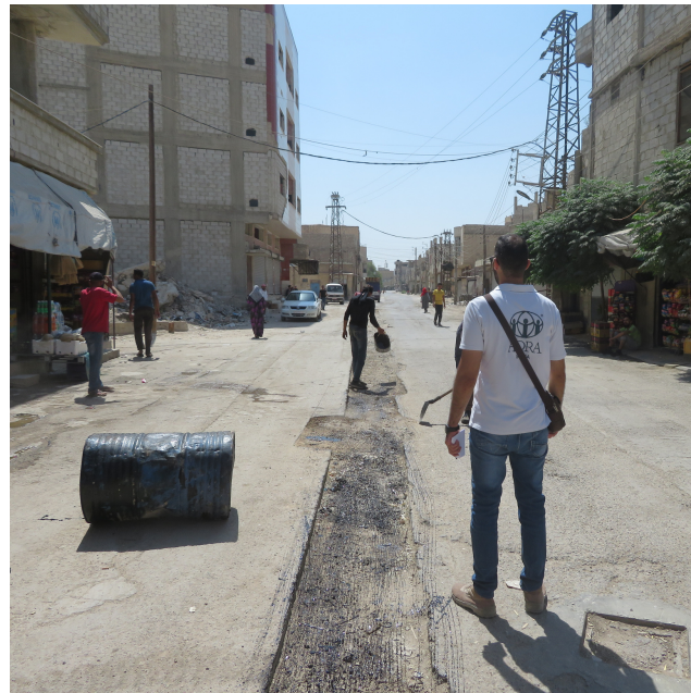
Asphalt layer after pipe rehabilitation September 2022
