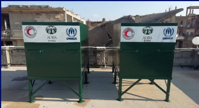
Above: Metal fuel tanks installed on the roof of the Hamedyah Health Center in Deir ez-Zour; Below/Right: Gate and fencing
