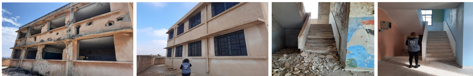
Above: Sakarja Middle School in Homs before and after rehabilitation
