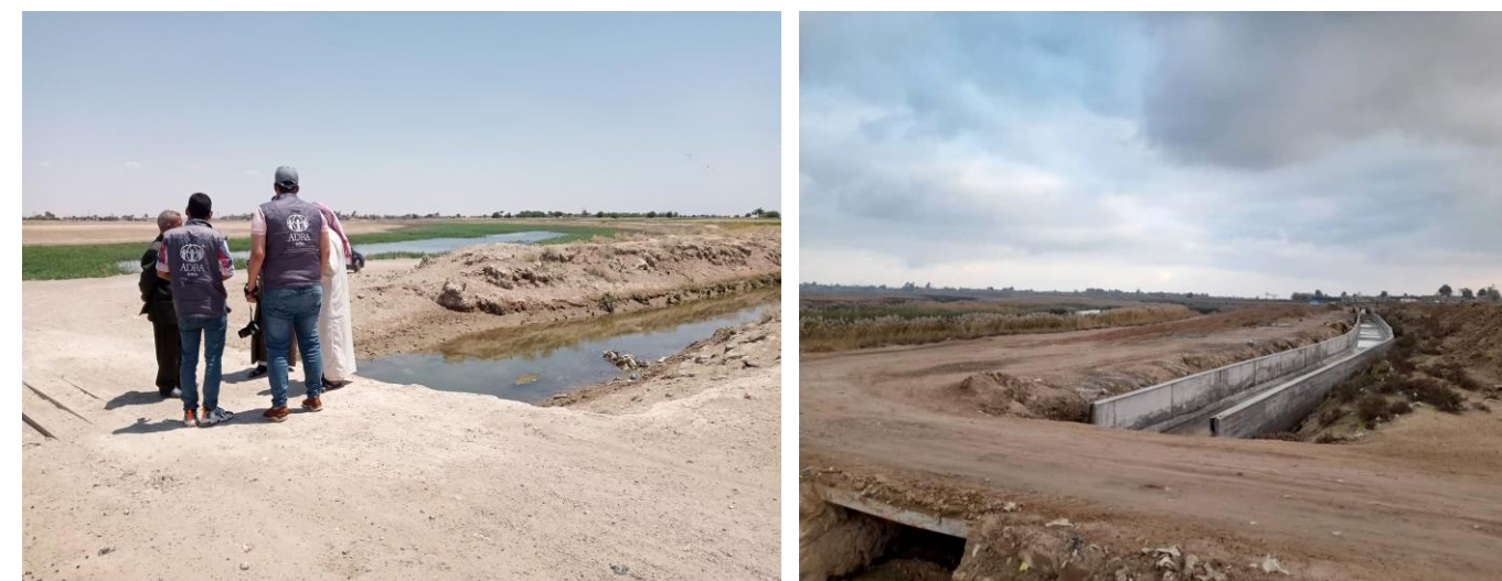
Before and after rehabilitation of the irrigation canal in Deir ez-Zour governorate
