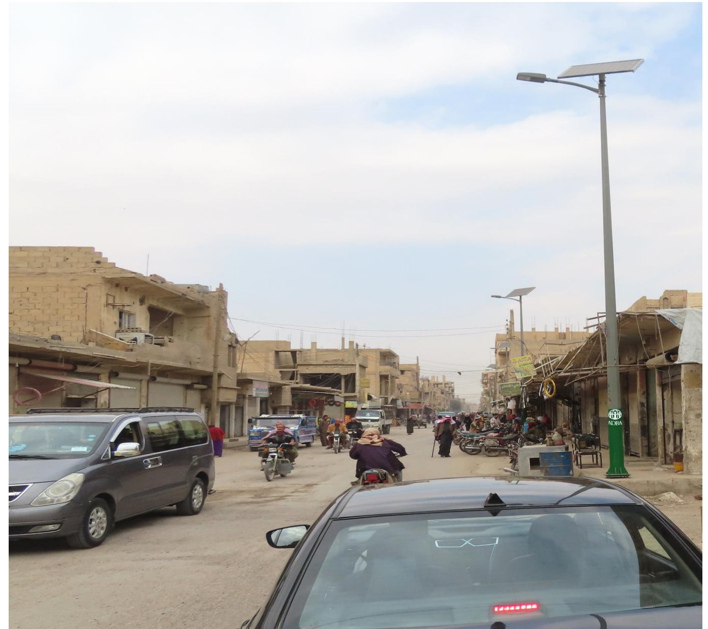
Installation of 55 streetlights (poles and solar panels) in Deir ez-Zour governorate
